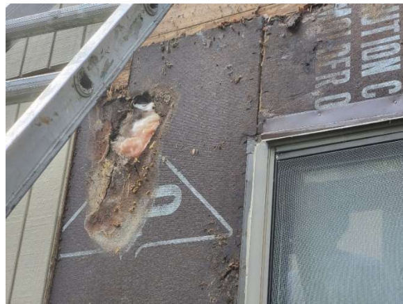
Photos 5 & 6: Wood framing exposed at floor line. Deteriorated fiberboard sheathing.
