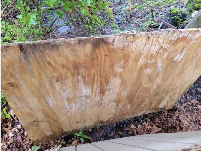
Photo 3 & 4: Wood T1-11 siding stained on back side. Severe deterioration at chimney
