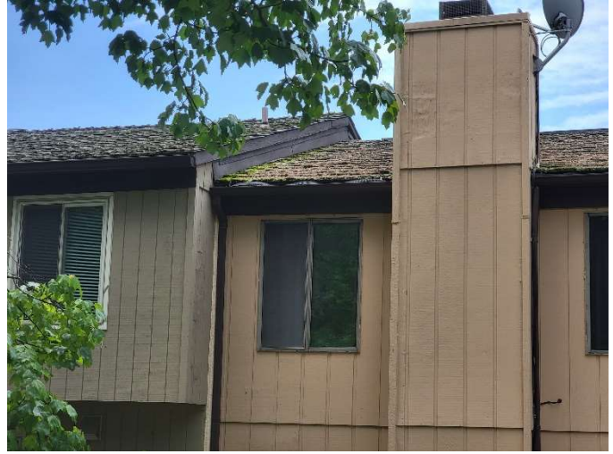
Photo 3 & 4: Wood T1-11 siding stained on back side. Severe deterioration at chimney
