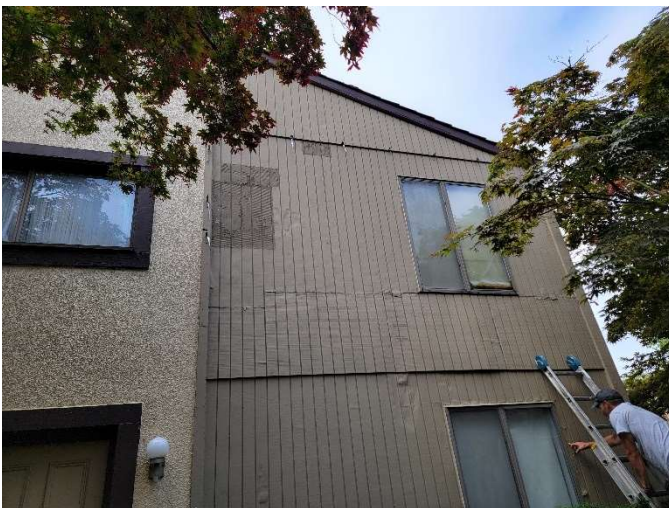
Photos 1 & 2: Wood T1-11 siding, visually bubbled/wavy where deteriorated.
