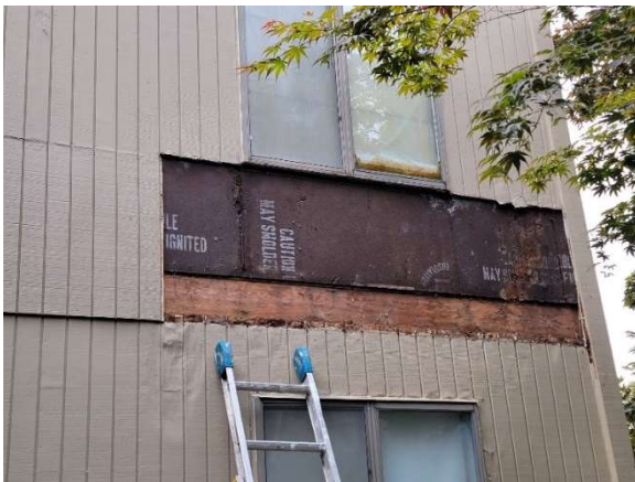
Photos 5 & 6: Wood framing exposed at floor line. Deteriorated fiberboard sheathing.
