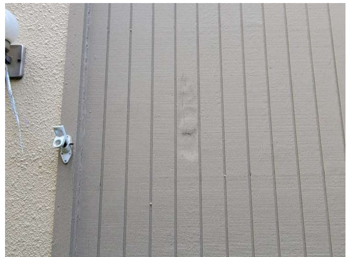
Photos 1 & 2: Wood T1-11 siding, visually bubbled/wavy where deteriorated.
